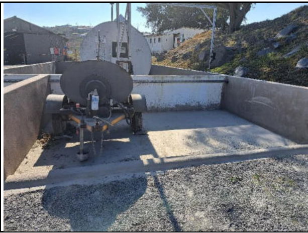
Diesel bowser parking area
