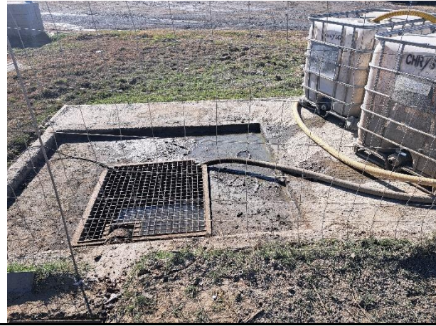
Oil sump pumped into the flow bins
