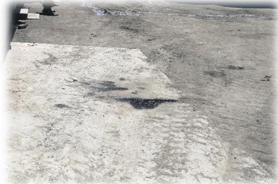
Fuell spillage due to the absense of driptrays.
