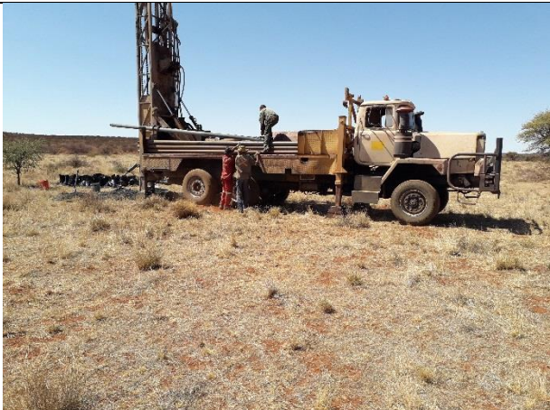
PERCUSSION DRILLING OF A BOREHOLE
