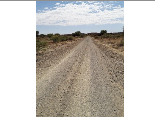
EXISTING ROAD INFRASTRUCTURE
