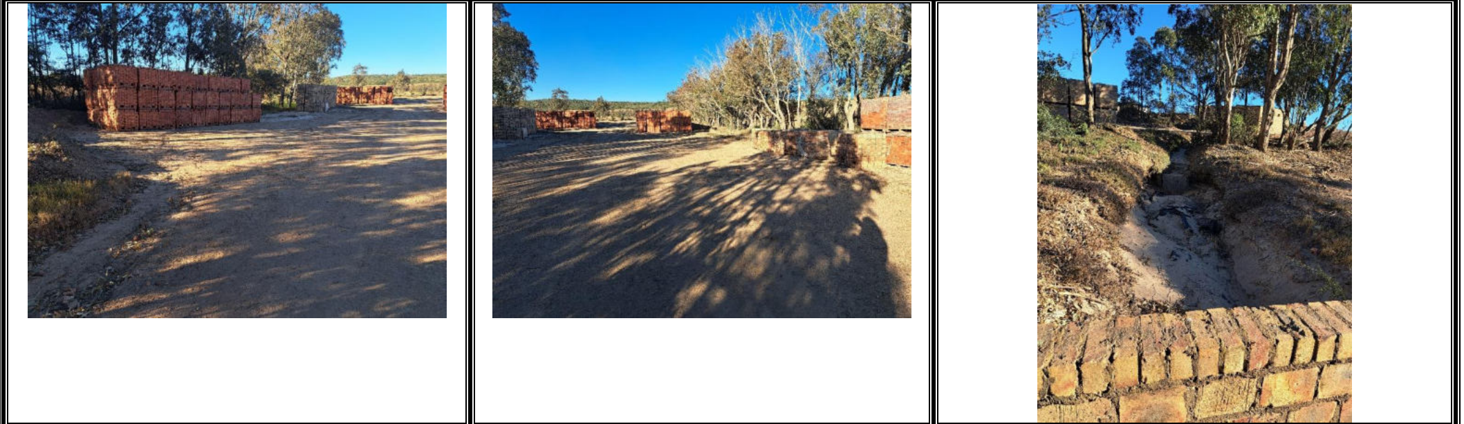
Brick storage area
