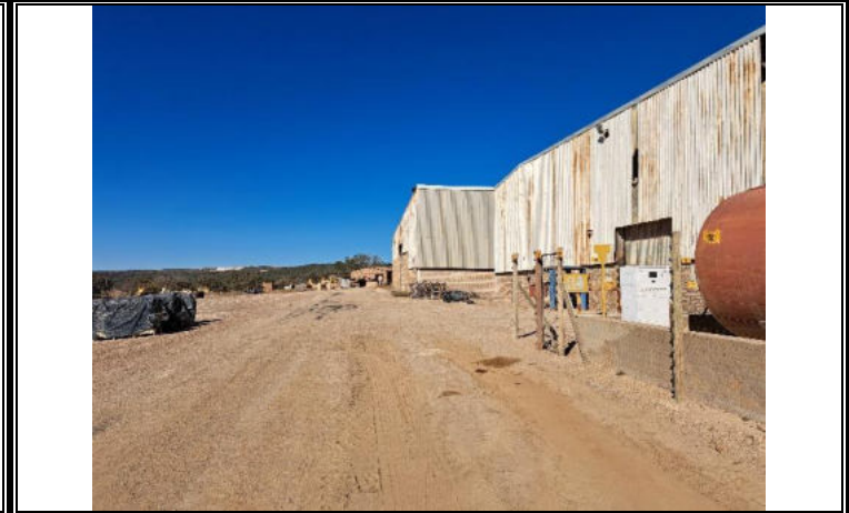
Tank to be placed in a bund
