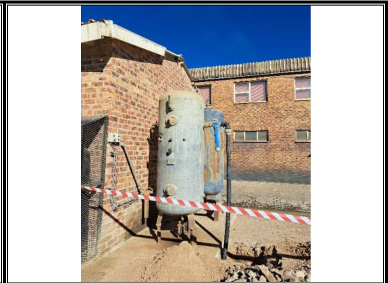
Tank to be placed in a bund
