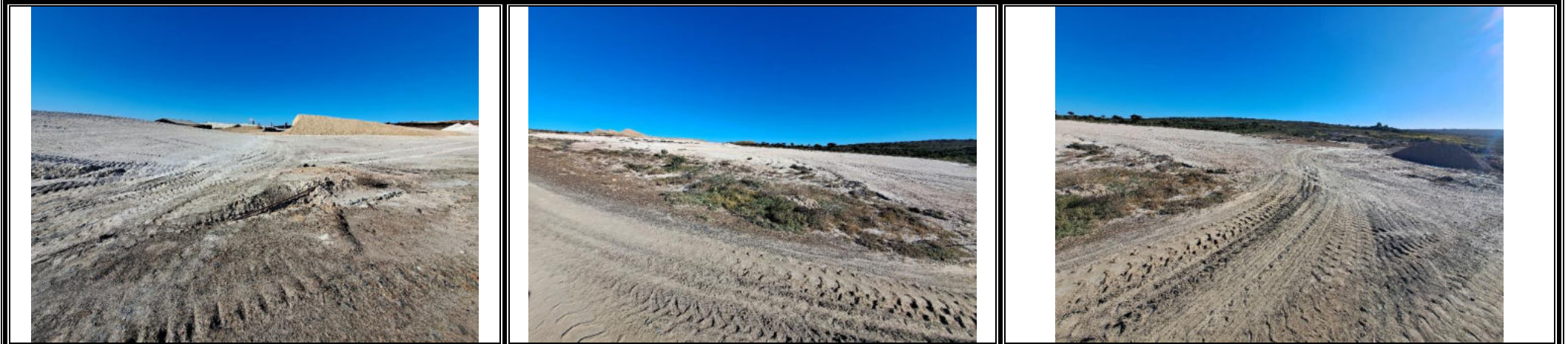
Stockpile areas neatly managed.
