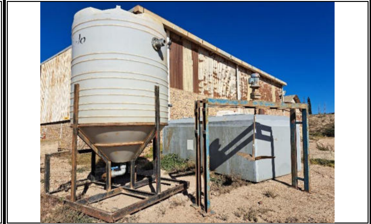
Tank to be placed in a bund
