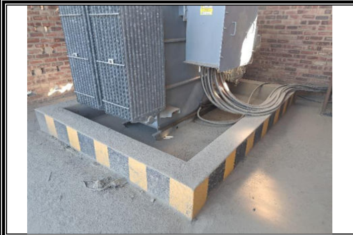
Bund at the processing plant
