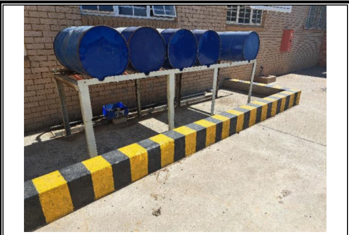
Bund at oil storage area
