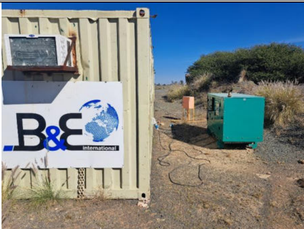
Drip trays and/or bunds to be added. Alternatively the equipment must be removed from site
