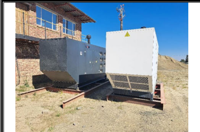
Bund to be installed around generators
