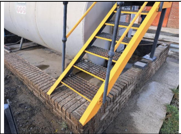
Diesel tank and bund wall
