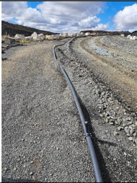
Sprayers installed to lessen dust generation
