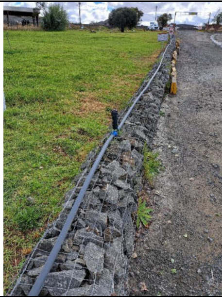
Sprayers installed to lessen dust generation
