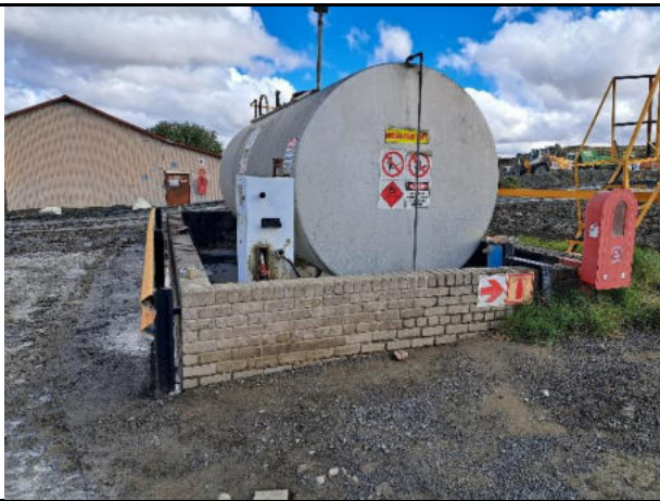
Diesel tank and bund wall
