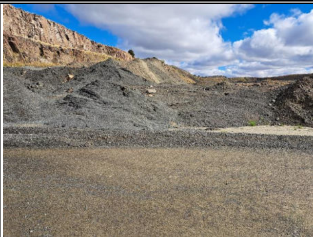
Sediment from the settling ponds used to rehabilitate the quarry
