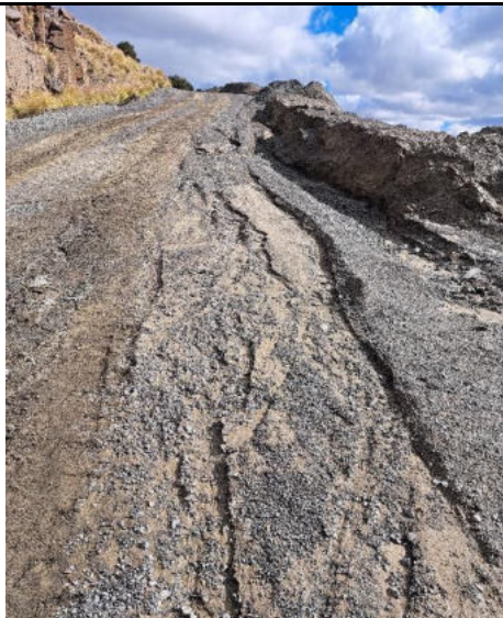
Sheet erosion due to rains – to be reinstated
