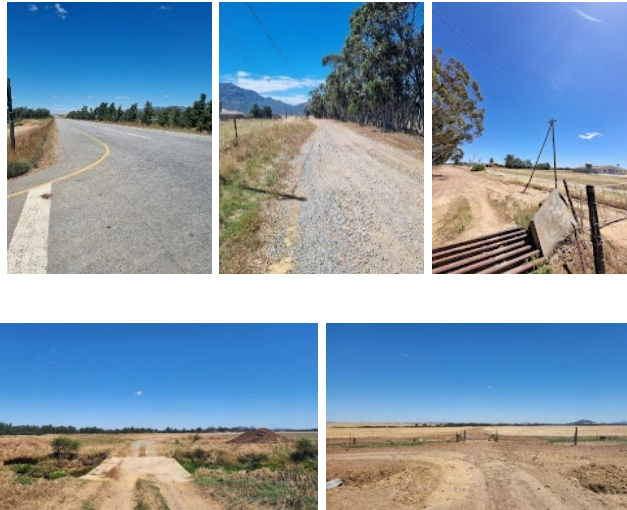
Figure 4: Photos showing the existing entrance into the mining area.
