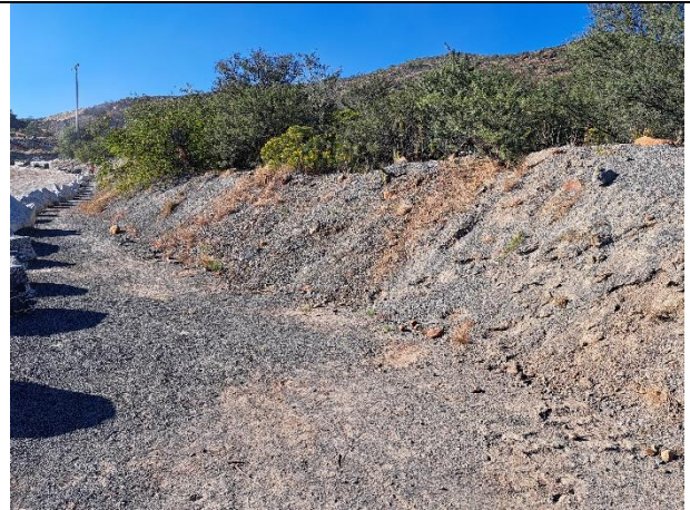
Stormwater berm
