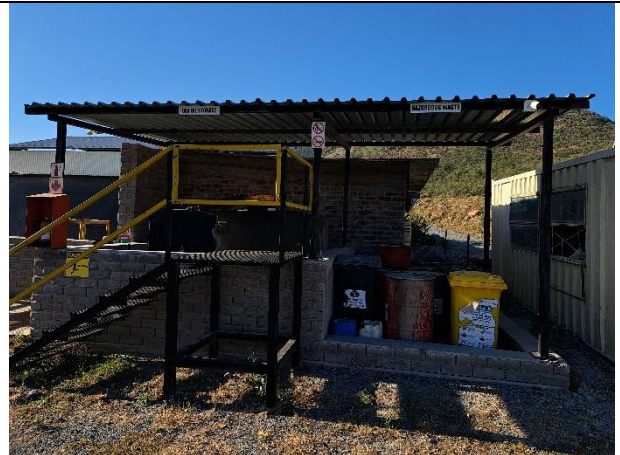
Used oil and hazardous waste storage area
