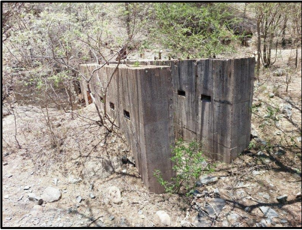
Figure 7.6. Foundation remains at RV003.
