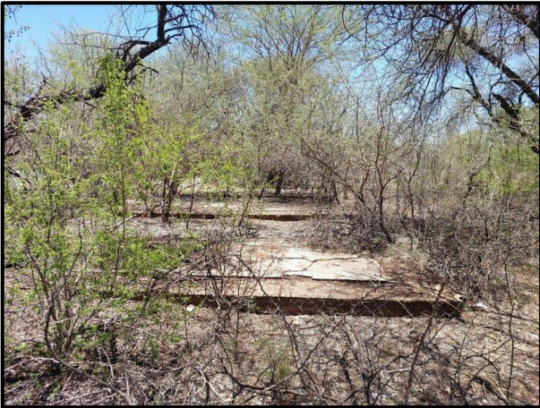
Figure 7.8. Foundation remains at RV004.
