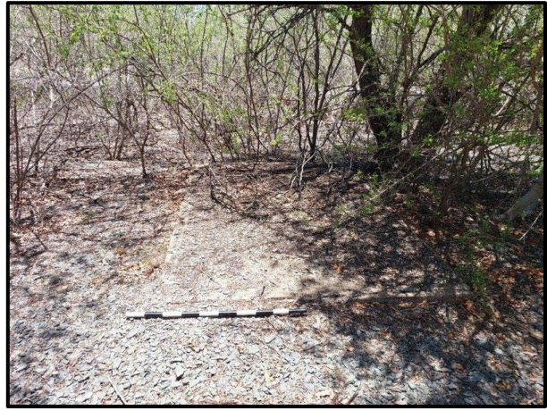
Figure 7.7. Remnants of a foundation at RV003.
