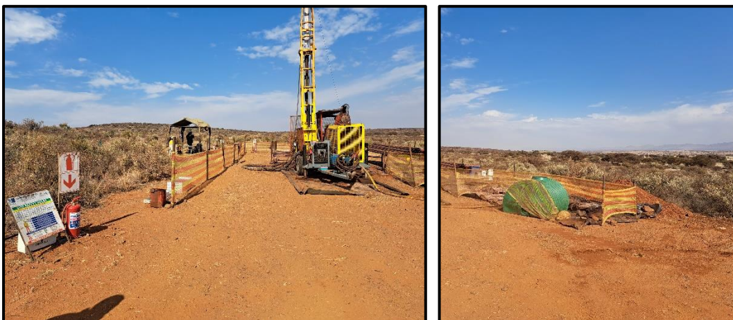
Figure 7: Example of a typical drill site.
