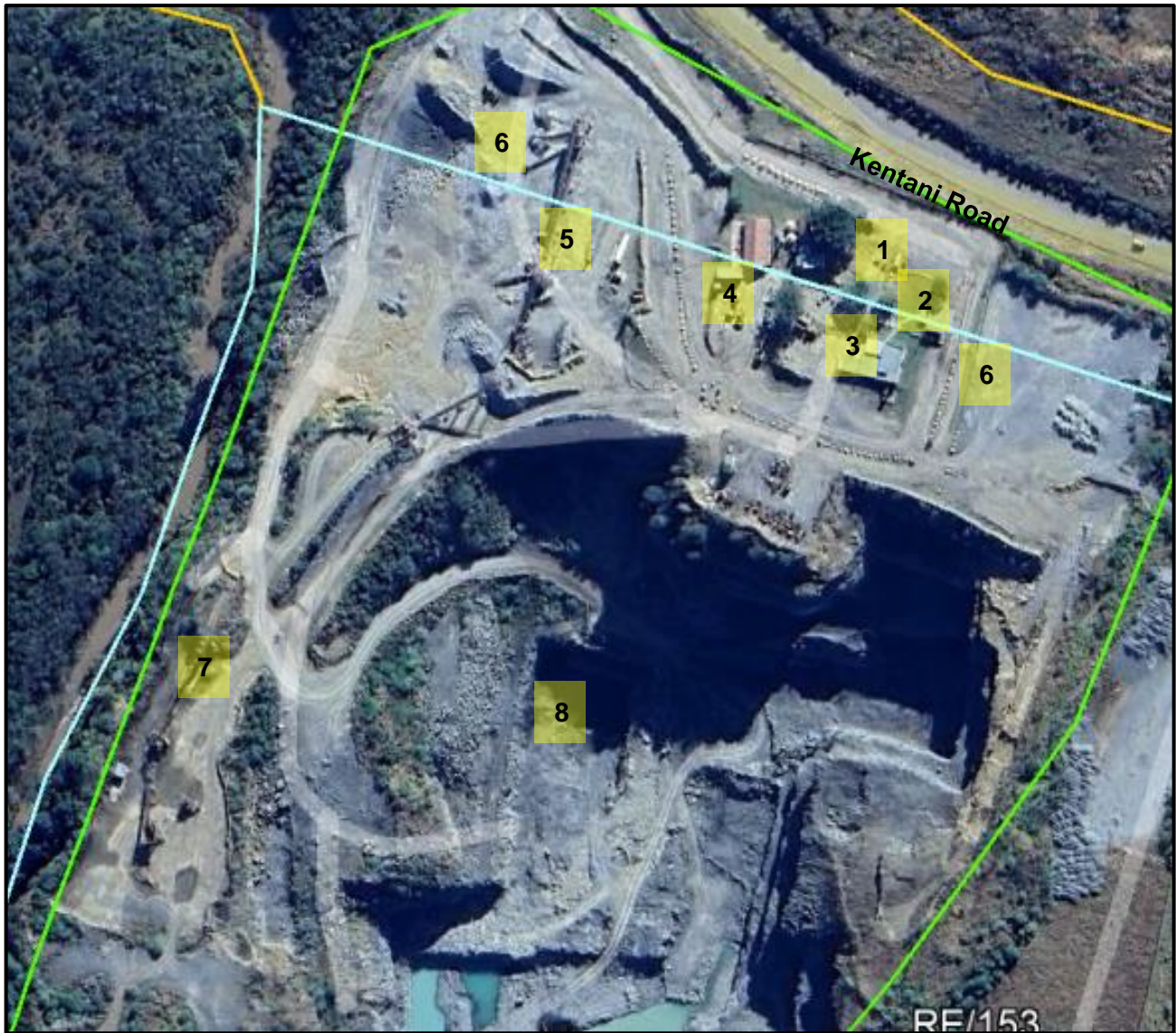
Figure 3: Satellite view of the various developed areas at Butterworth Quarry (image obtained from Google Earth)
