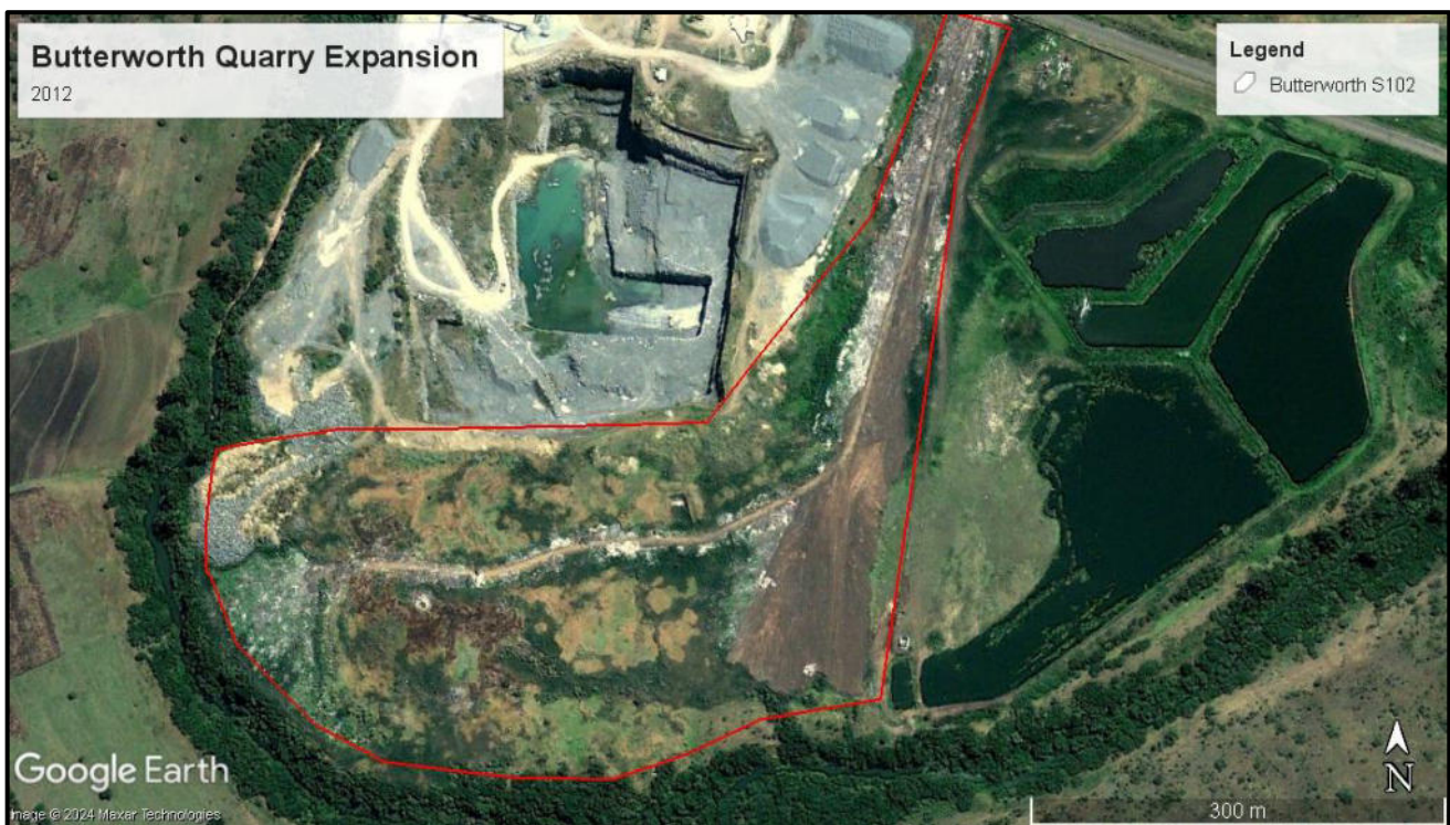
Figure 3.2. 2012 Google image indicating additional dumping in the western section of the Project area. Mining activities has expanded especially to the west, and the road and surrounding areas have been cleared.
