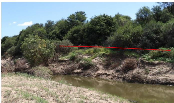
View of the upper zone of the riverbank. The upper zone is most easily discerned by dense riparian thicket and a gradual slope but which increases substantially into the lower zone. The riverbank will be affected by sand excavation, access roads and pump infrastructure.
